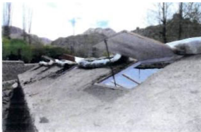
Picture 47 - Day view of roof ventilation
